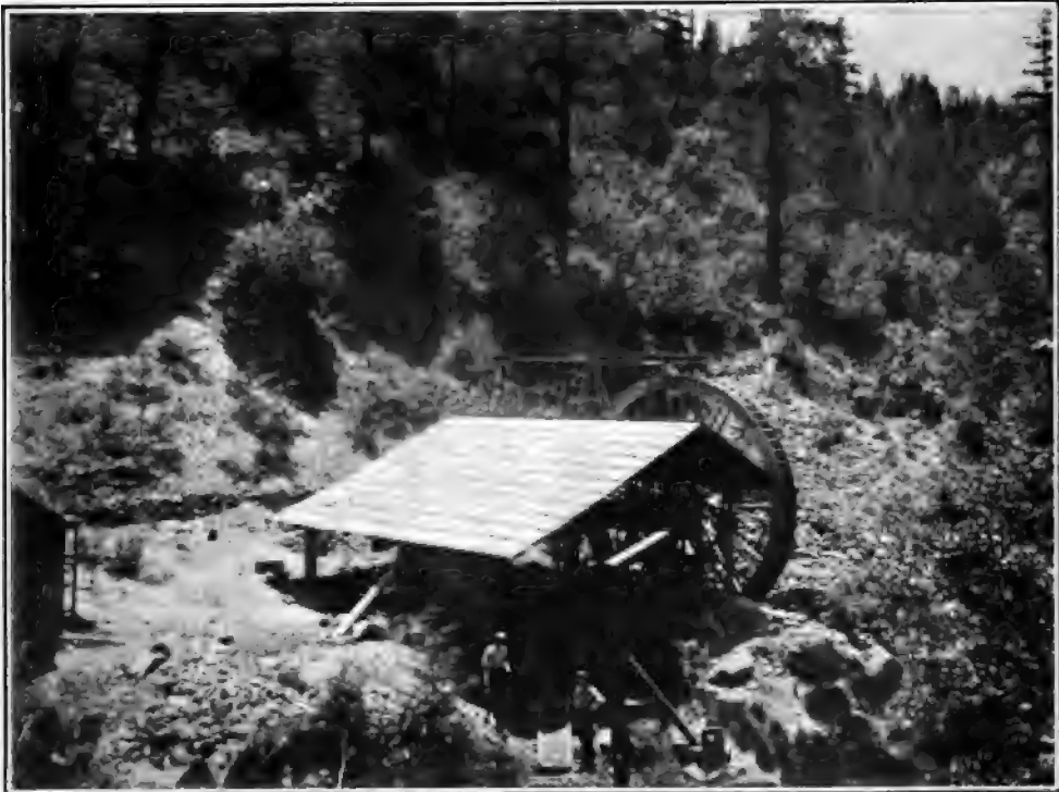
ARASTRA, NEAR DELTA, USED IN GRINDING AND AMALGAMATING ORE
